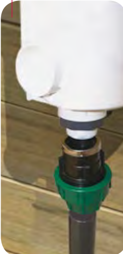
Rigid descending pipe under the skimmer
